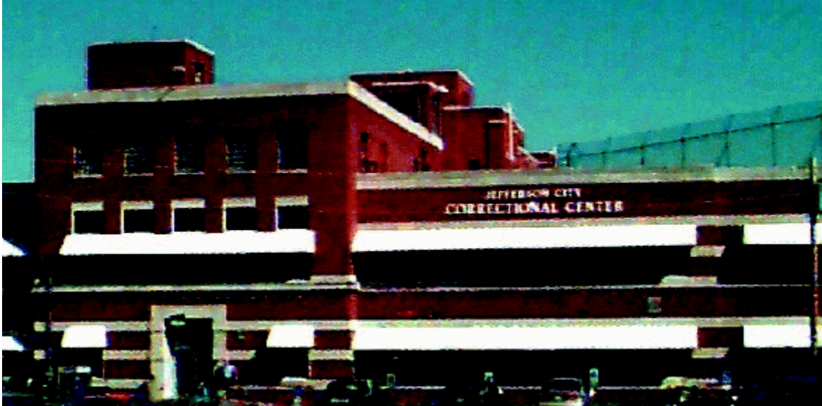
JCCC Administration Building
