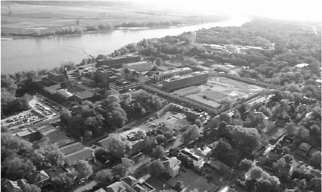
Correctional Center property from South West
